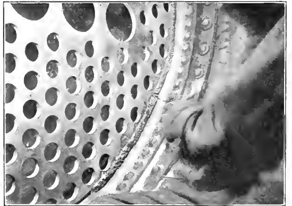
Welding a Front Tube Sheet
